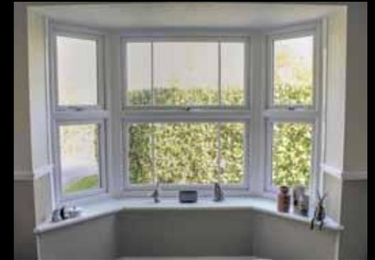
The below example clearly shows how dummy casements help to achieve equal sight lines. The left image shows opening sashes either side of a fixed pane.
