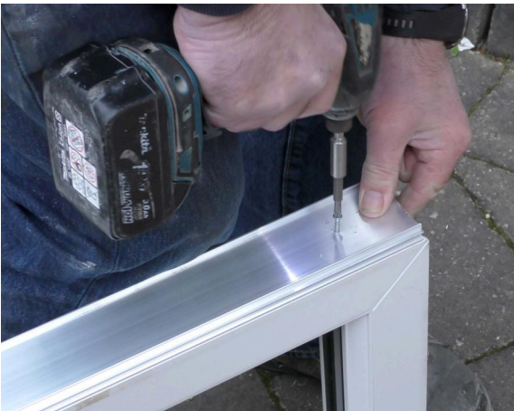
Measure, cut and fix the coupler to the light.
