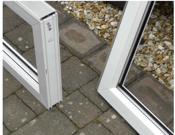
Make sure the couplers are positioned the correct side to connect with the door frame and the drainage holes are positioned at the bottom and at the external face of the light.
