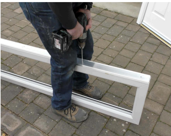
Insert fixing holes to the coupler every 600 millimetres.
